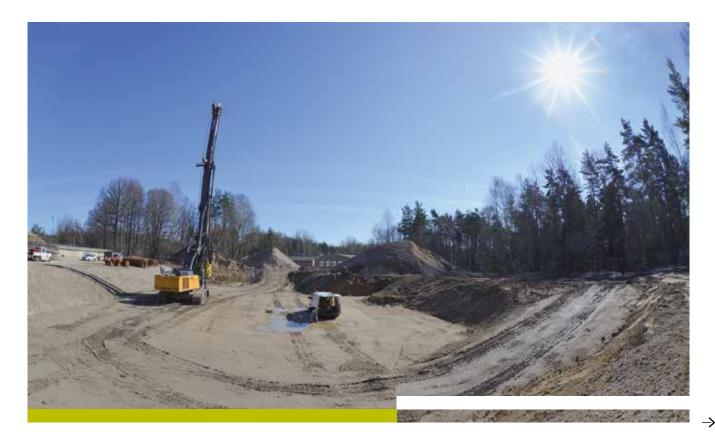
STILL UNDER CONSTRUCTION: The drill is waiting to dive 22 meters deep and lay the deep foundation for the dynamo, which weighs tons. Photo: Matthias Rietschel
