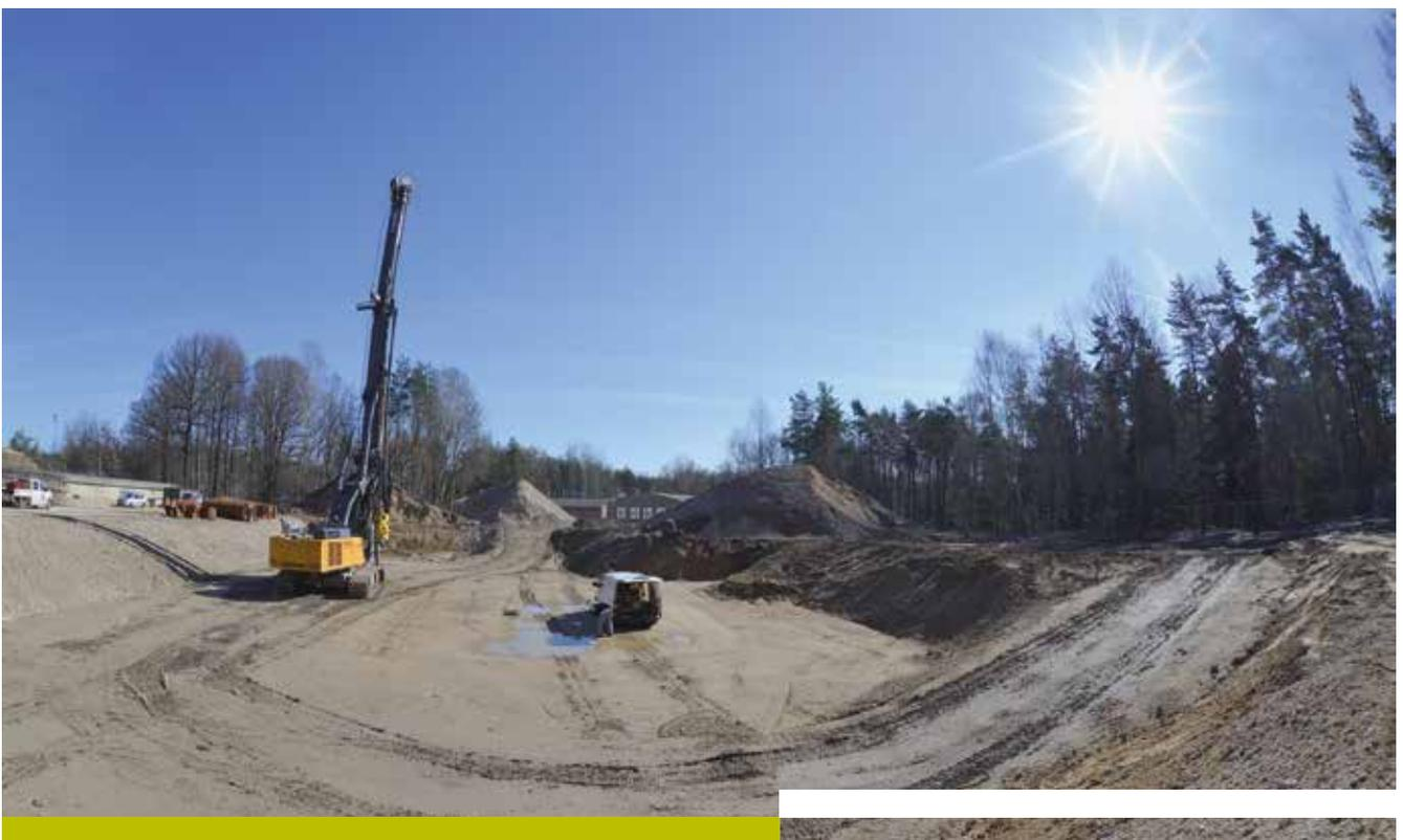
**STILL UNDER CONSTRUCTION:** The drill is waiting to dive 22 meters deep and lay the deep foundation for the dynamo, which weighs tons.
