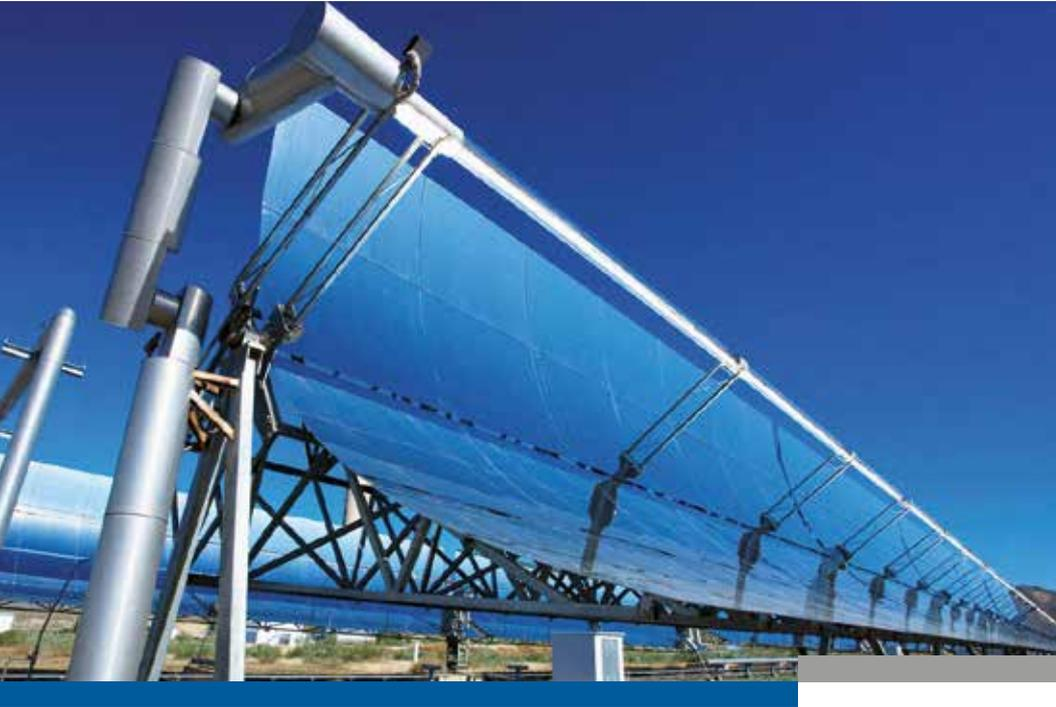
**A DIFFERENT KIND OF POWER PLANT:** Parabolic trough power plants use focusing mirrors to concentrate sunlight onto an absorber tube. The heat energy that is captured within the tube is then used to produce steam to power a turbine. Photo: DLR
