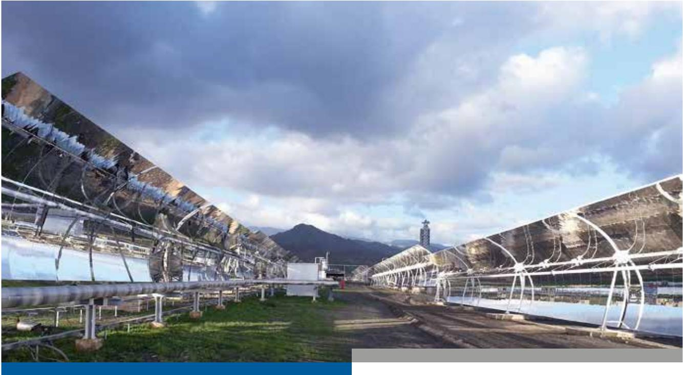
**WITHOUT ANY LOSSES:** At the DUKE test facility, steam is generated directly inside the parabolic troughs' tubes for subsequent power production. Photo: DLR
