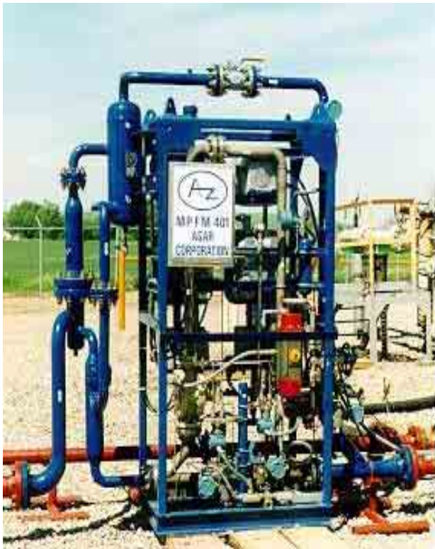
Fig. 2. Multiphase flow meter "Agar MPFM"
