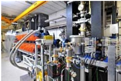
TELBE-facility at HZDR Source: HZDR / Frank Bierstedt
