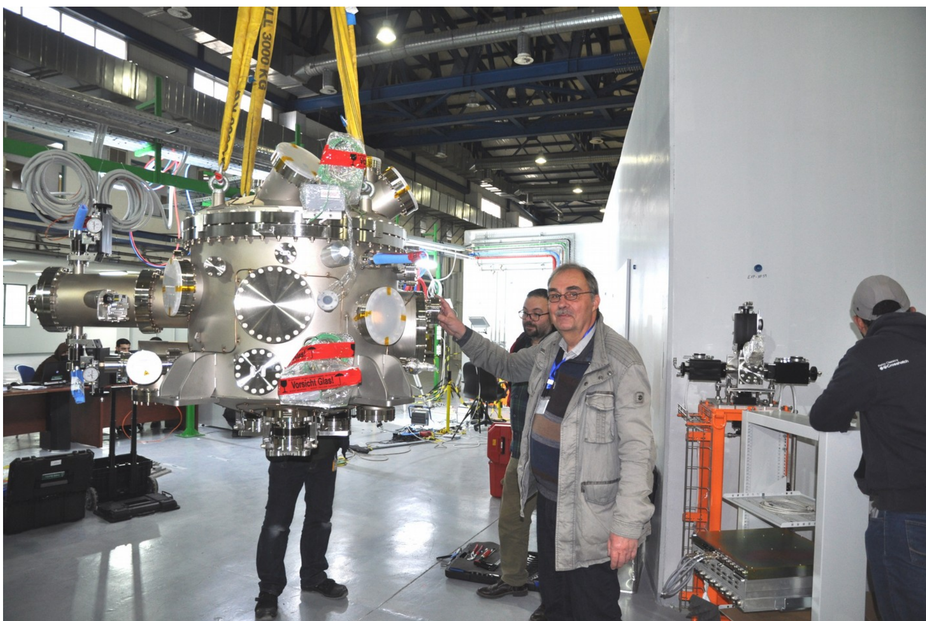
moving PGM chamber into place
